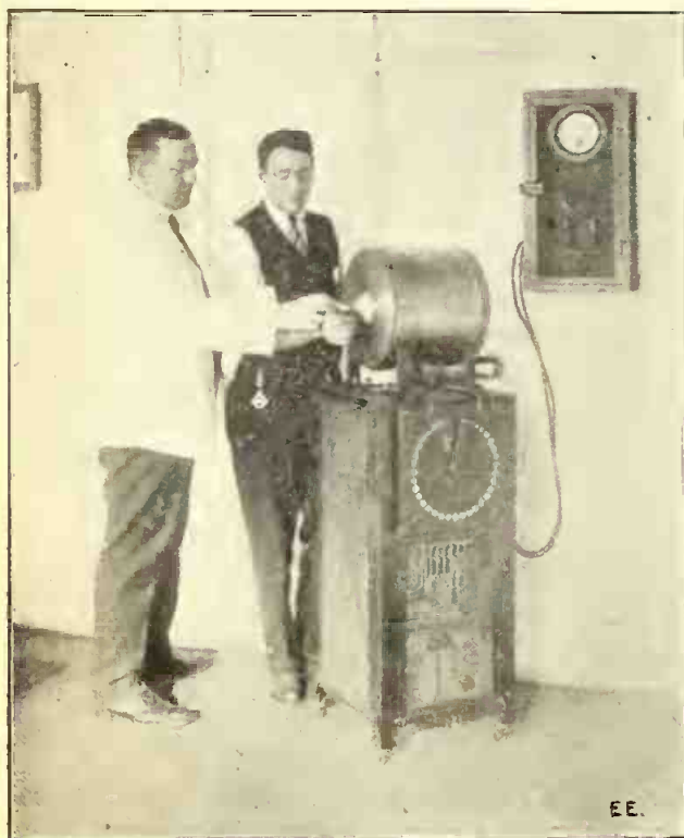
Powerful Electromagnet Draws Iron or Steel Chips From Fingers, Eyes, Etc.
